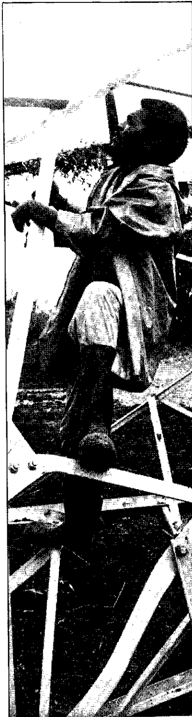
Electrical worker repairs MNR sabotaged pylon
