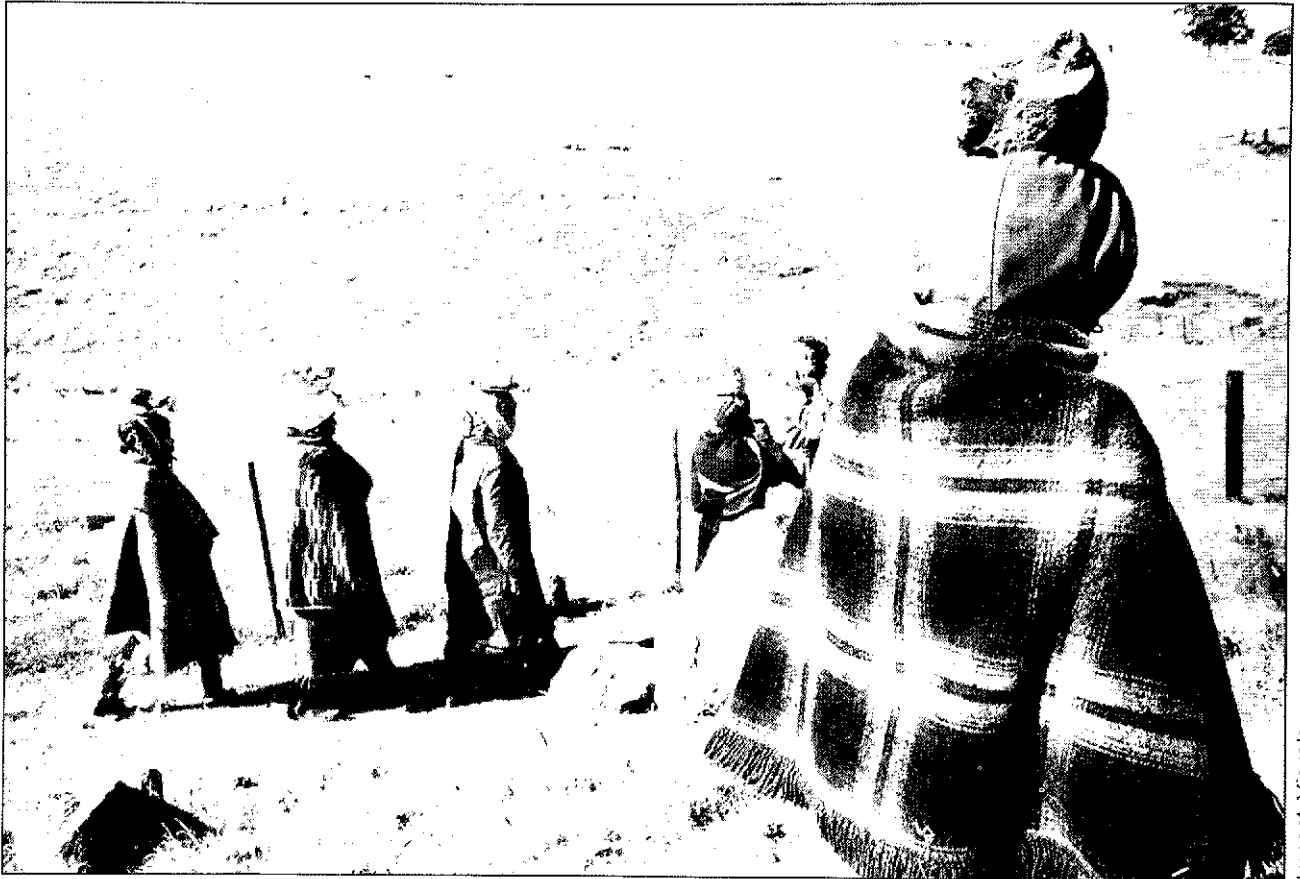
Women road construction workers carry rocks to repair a dirt road in the Transkei
