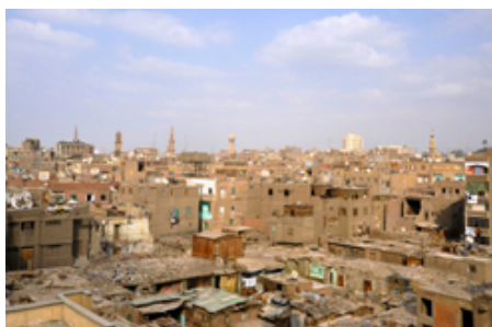
Over 6 million people living in perilous conditions: one of Cairo's many slums (foreground)
