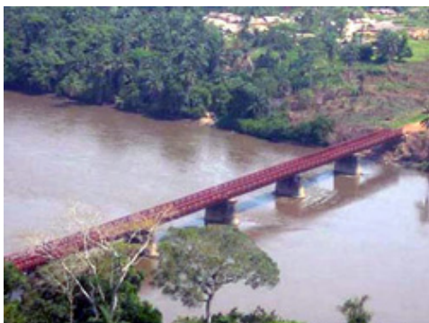
A bridge near Bafwasende, DRC: much of the country's infrastructure is in an advanced state of disrepair.
